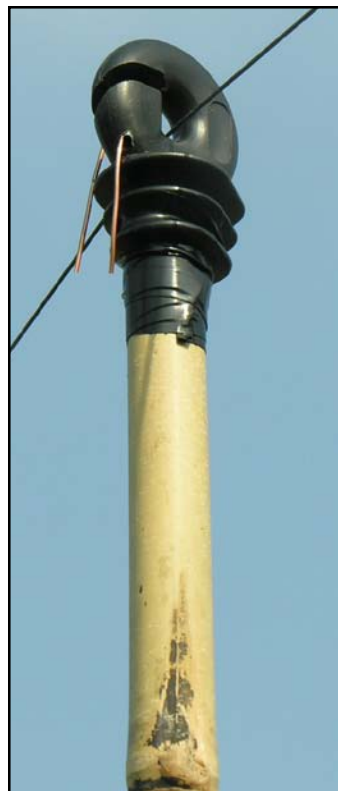
Fig 7-106 — A 2.4 meter long bamboo stick can be used to support the Beverage wire. ON4UN uses electric fence insulators on top of the bamboo sticks (see text).
