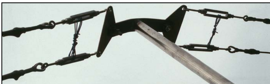
Fig 13-11 — Details of the tension-equalizing system at the top of the support mast, where the two boom-support trusses are attached. The triangular-shaped plate can rotate freely around the 10-mm bolt, which serves to equalize the tensions in the two guy wires. See text for details.
