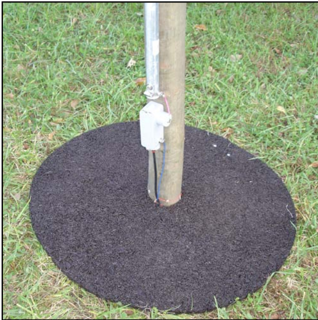
Fig 7-57 — To prevent having to remove the grass and weeds that cover the base of verticals, Charlie, NØTT, slipped a disk made of roofing shingles over the wooden support poles at his Nine Circle array. Nice and tidy.
