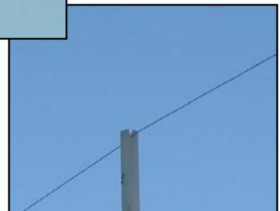
Fig 7-107 — A piece of good quality plastic tube slid over a rebar driven into the ground makes a good and strong support. A slit at the top captures the wire and lets it slide freely (seen at K9DX and W8JI).
