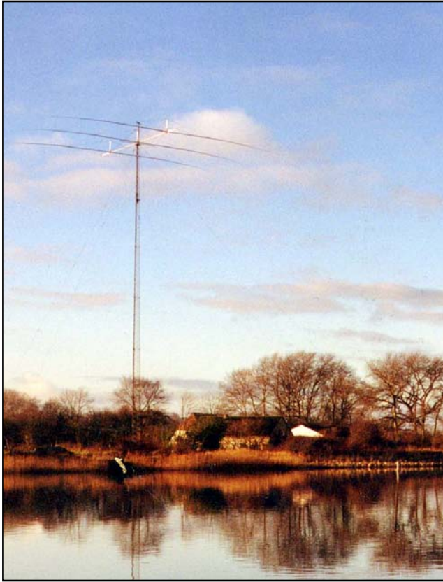
Fig 13-30 — OZ8BV's 3-element full-size 80-meter Yagi atop of his 48-meter tower on the Danish Baltic sea shore (in the 1990s)
