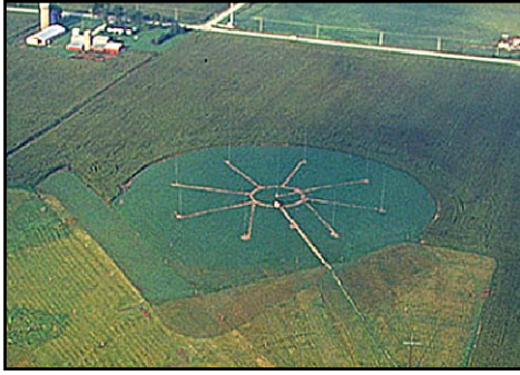
Fig 11-156 — Aerial picture of the K9DX Nine Circle array as constructed by John, K9DX. The circular array, including the radials that extend 40 meters from the array itself, has a diameter of 208 meters (two soccer fields long!). The thick stripes are the feed line trenches that had not grown over when the picture was taken.
