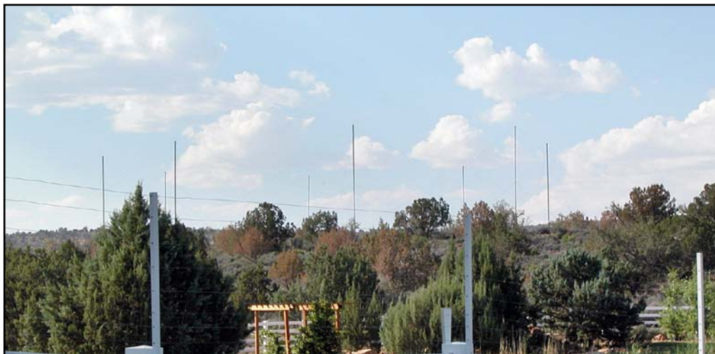
Fig 7-60 — At N7JW's QTH in St George, Utah, we see the eight elements of his Eight Circle array on top of a ridge. This array consists of two side-by-side 2-element parasitic vertical groups, spaced approximately 94 meters. Similar to W8JI's Eight Circle in concept, it is switchable in eight directions. The main difference from W8JI's Eight Circle is that N7JW's antenna is a transmit array as well.
