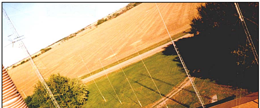
Fig 13-53 — Bird’s eye view from the driven element of the 160-meter array at KØHA. The first director, on the left of the picture, is hiding from the second director. On the right a line of elements for the 80-meter array aims at Europe. It also appears that Bill enjoys some of the best ground conductivity around. No wonder he’s loud!
