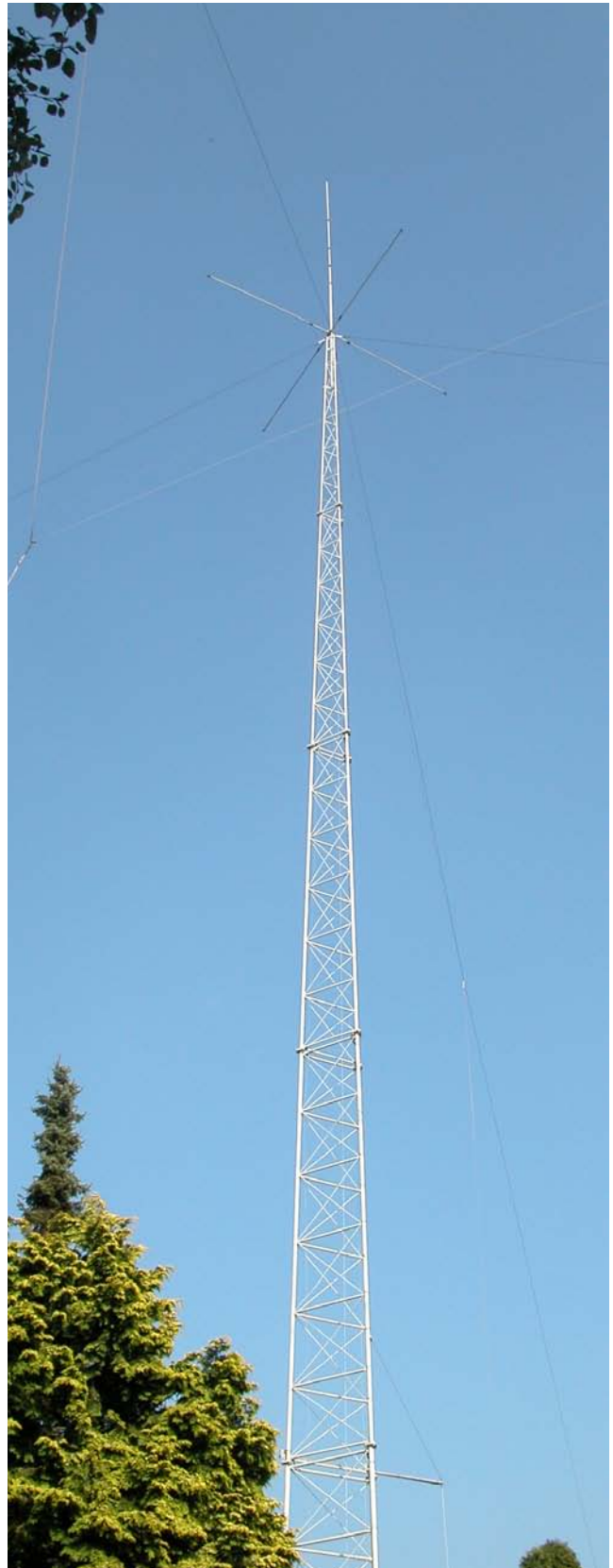
Fig 9-74 — Self-supporting 39.5-meter \lambda/4 vertical for 160 meters at ON4UN. The base is 1.8 meters wide and the tower tapers to just a few inches at the top. The tower is shunt fed with a gamma match and also serves as a support for an 80-meter Four Square array made of \lambda/4 verticals, supported from sloping catenary lines running from the 160-meter tower.
