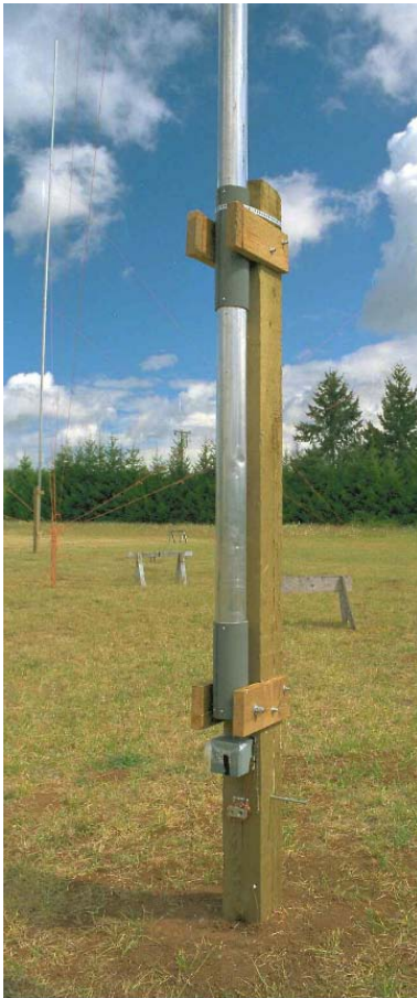
Fig 9-68 — Base of one of the irrigation- pipe 80-meter verticals constructed by K7EM.
