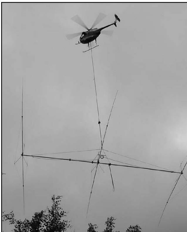
Fig 13-42 — OH2BH's 3-element 80-meter Yagi was flown by helicopter from the assembly area to the tower, which is in the middle of the woods about 1 km away.
