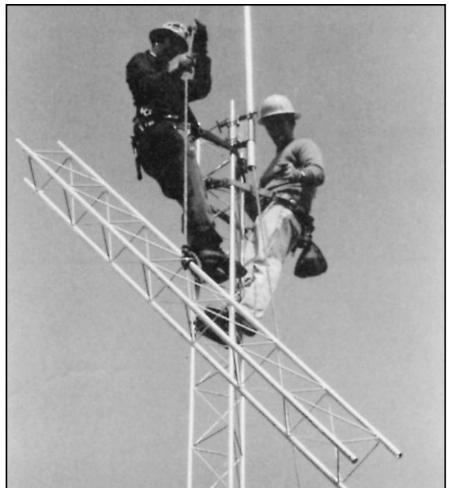
Fig 5—The assembly of tower sections is made simple when a gin pole is used to lift each one into position. Note that the safety belts of both climbers are fastened below the pole, thereby preventing the strap from slipping over the top section. (Photo by K1WA)
