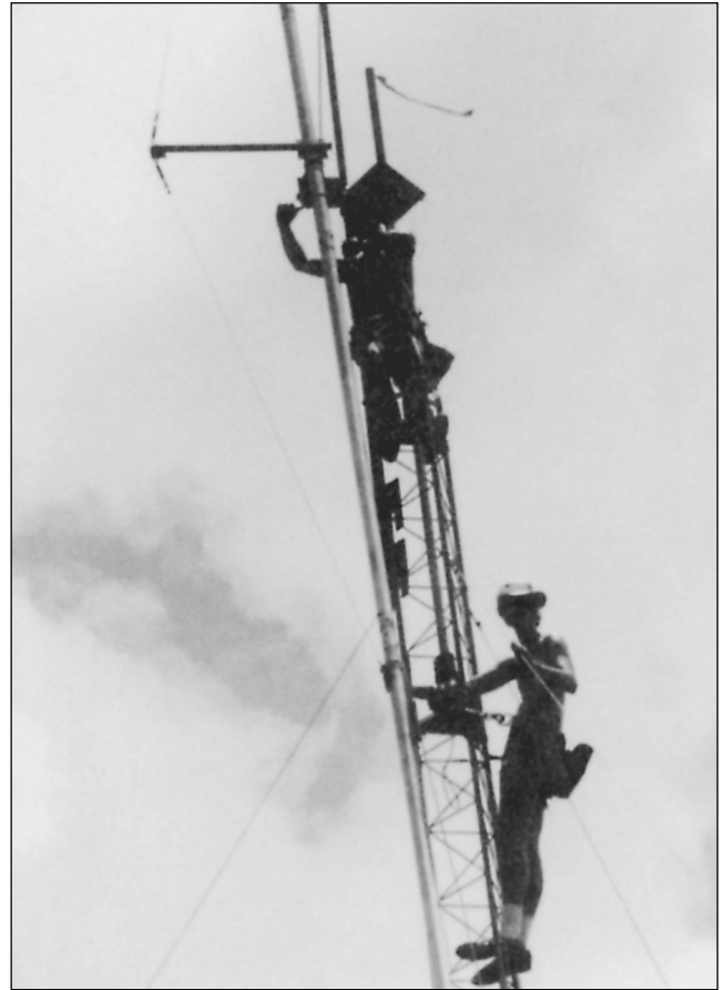
Fig 39—Working at the 70-foot level. A gin pole makes pulling up and mounting the boom to the boom plate a safe and easy procedure.
