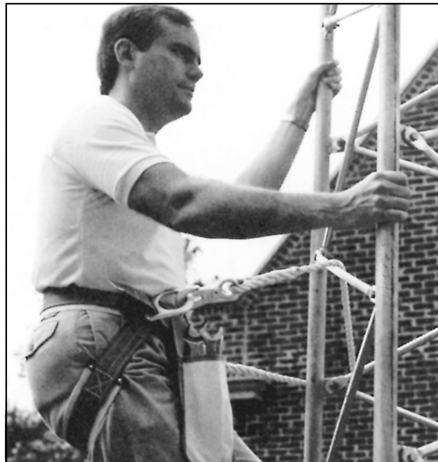
Fig 7—Mark Wilson, K1RO, shows the proper way to attach a safety hook, with the hook opening facing away from the tower. That way the hook can't be accidentally released by pressing it against a tower leg.
