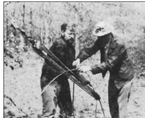
Fig 22—Proper tension can be placed on the guy wires with the aid of a block-and-tackle system. (Photo by K1WA)
