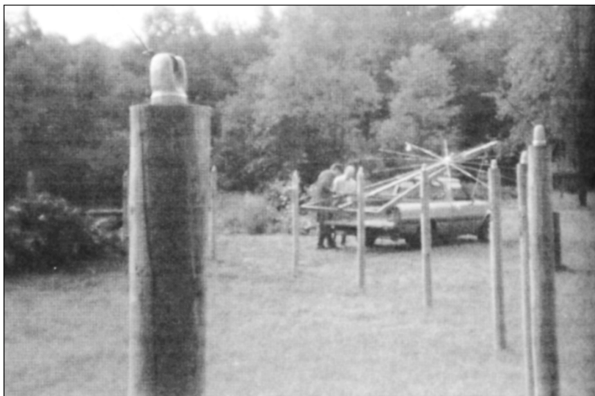
Fig 49—Photo showing some of the fence posts used to hold individual cone wires to keep them off the ground and out of harm's way. The truck in the background is carting away the A-frame discone for installation at KA8UNO's QTH.
