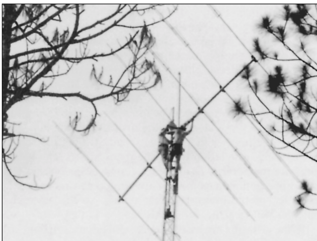
Fig 41—The U bolts securing the short pipe to the mast plate are loosened and the boom is turned to a horizontal position. This puts the elements in a vertical plane. Then the pipe U bolts are tightened and pinning bolts secured. The boom U bolts are then loosened and the boom turned axially 90°.
