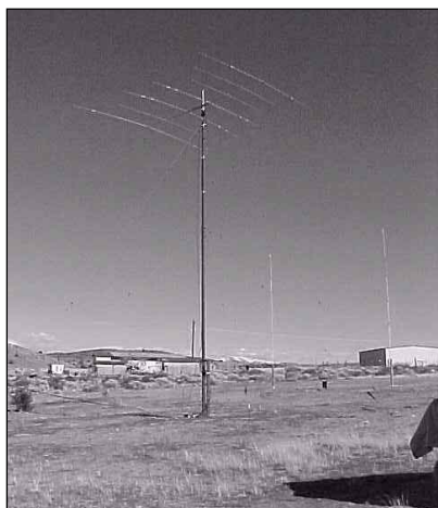
Fig 18 —Installation of surplus AB-577 tower with triband at 45 feet at K7NV. (Photo by Kurt Andress, K7NV)
