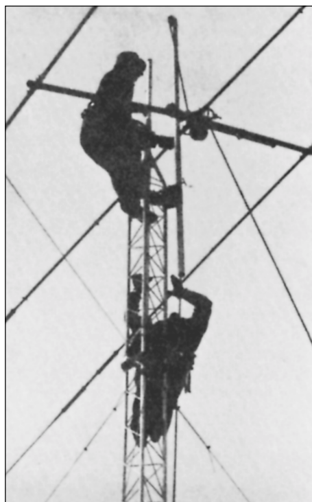
Fig 21—A gin pole is helpful in positioning antennas and tower sections. The ground crew holds the weight of the assembly with a heavy rope, making tower work safer and less tiring. (Photo by Dave Pietraszewski, K1WA)
